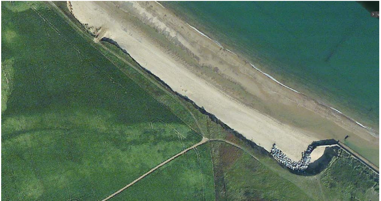
Figure 17. Access ramp (top right) created for construction of rock wall at south-eastern end of the beach (bottom left) in approximately 2010. Bing Maps.
