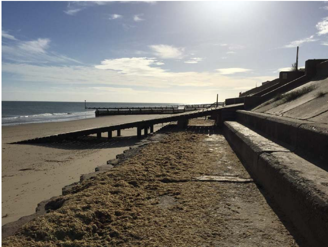
Figure 17. Timber beach access ramp at Bacton Gap.
