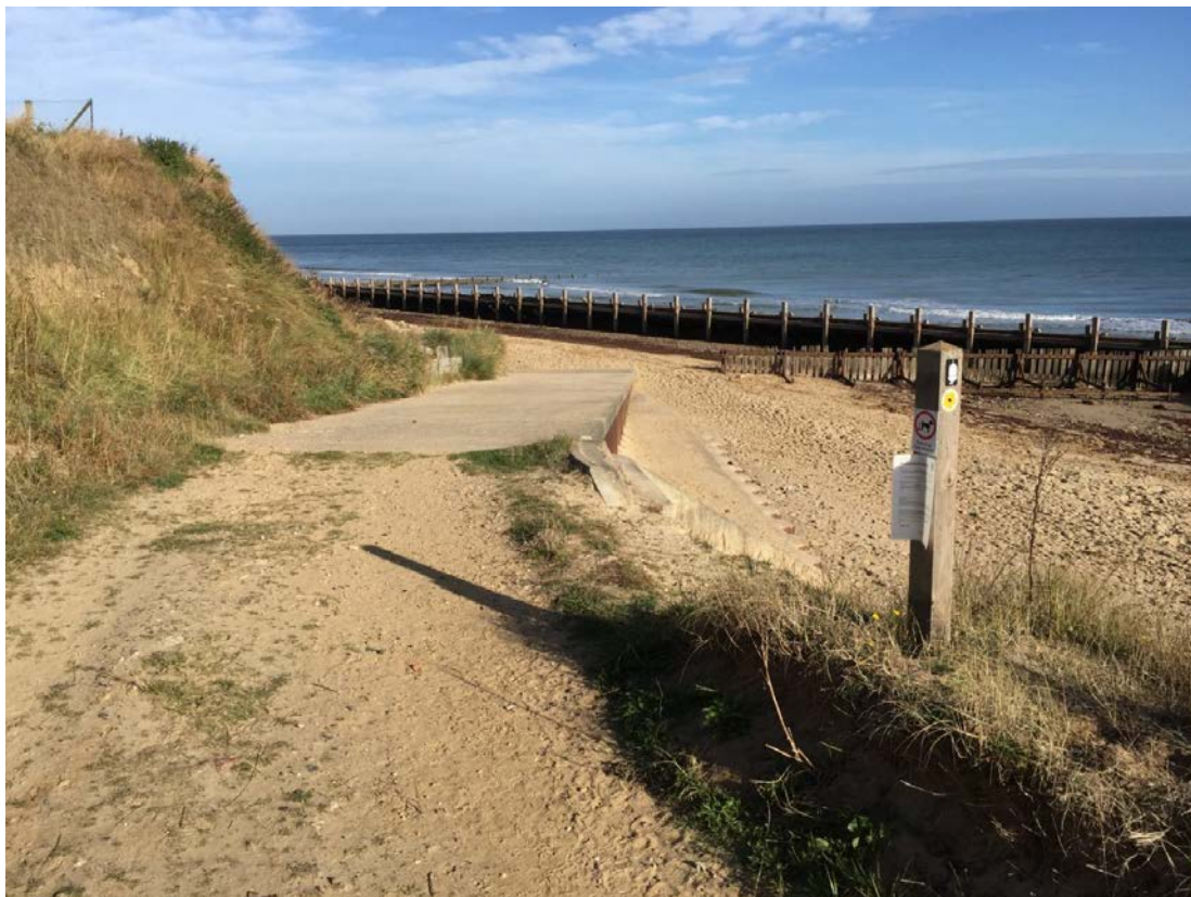
Figure 16. Low angle access ramp to the beach at the northwestern corner of the field. The location is at the far end of the track in the previous photograph. Design 1 passes beneath this view point.
