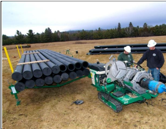
Figure 29. Typical setup of PE butt fusion welder
