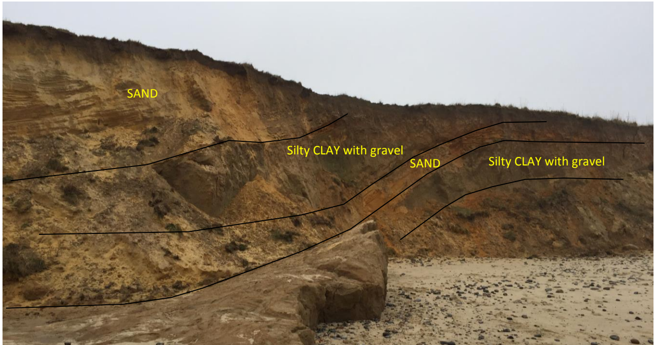
Figure 6. Photograph showing the north-western margin of the subsidence basin. The lower left of the photograph shows the lower silty CLAY with gravel layer within the basin approaching a near horizontal attitude. The right of the photograph shows the horizontal strata in the unaffected zone. The centre of the photograph shows inclined strata along the margin of the subsidence area.
