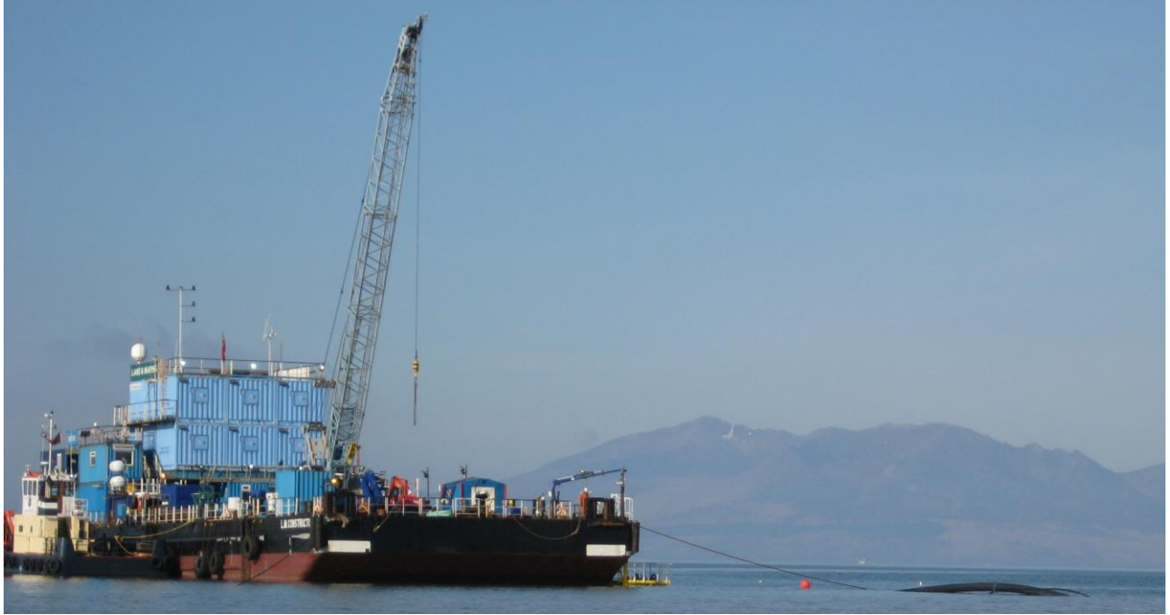
Figure 31. Large barge with four point anchoring. On the right hand side of the barge the duct can be seen being pulled into the HDD. The water depth is approximately 4m.
